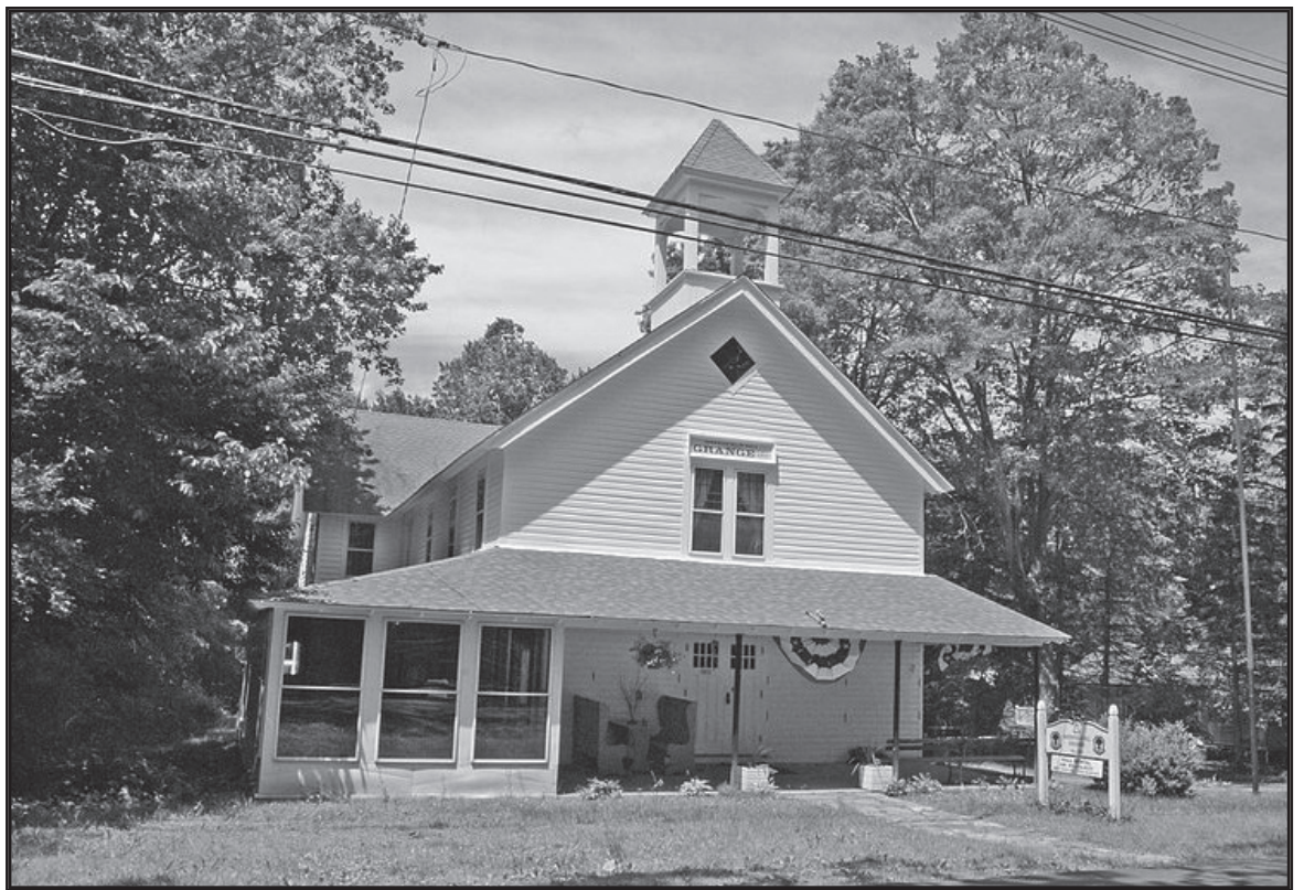
Greenfield Hill Grange hall as it stands today. The large flag pole on the roof is now gone but many of the distinguishing features are still there. Over time a porch and an addition to the back of the hall have been constructed.
