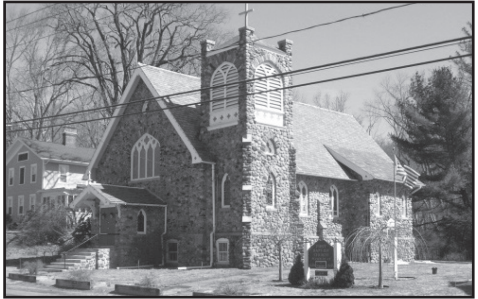
The former St. Peter's Episcopal Church in Plymouth, CT.
